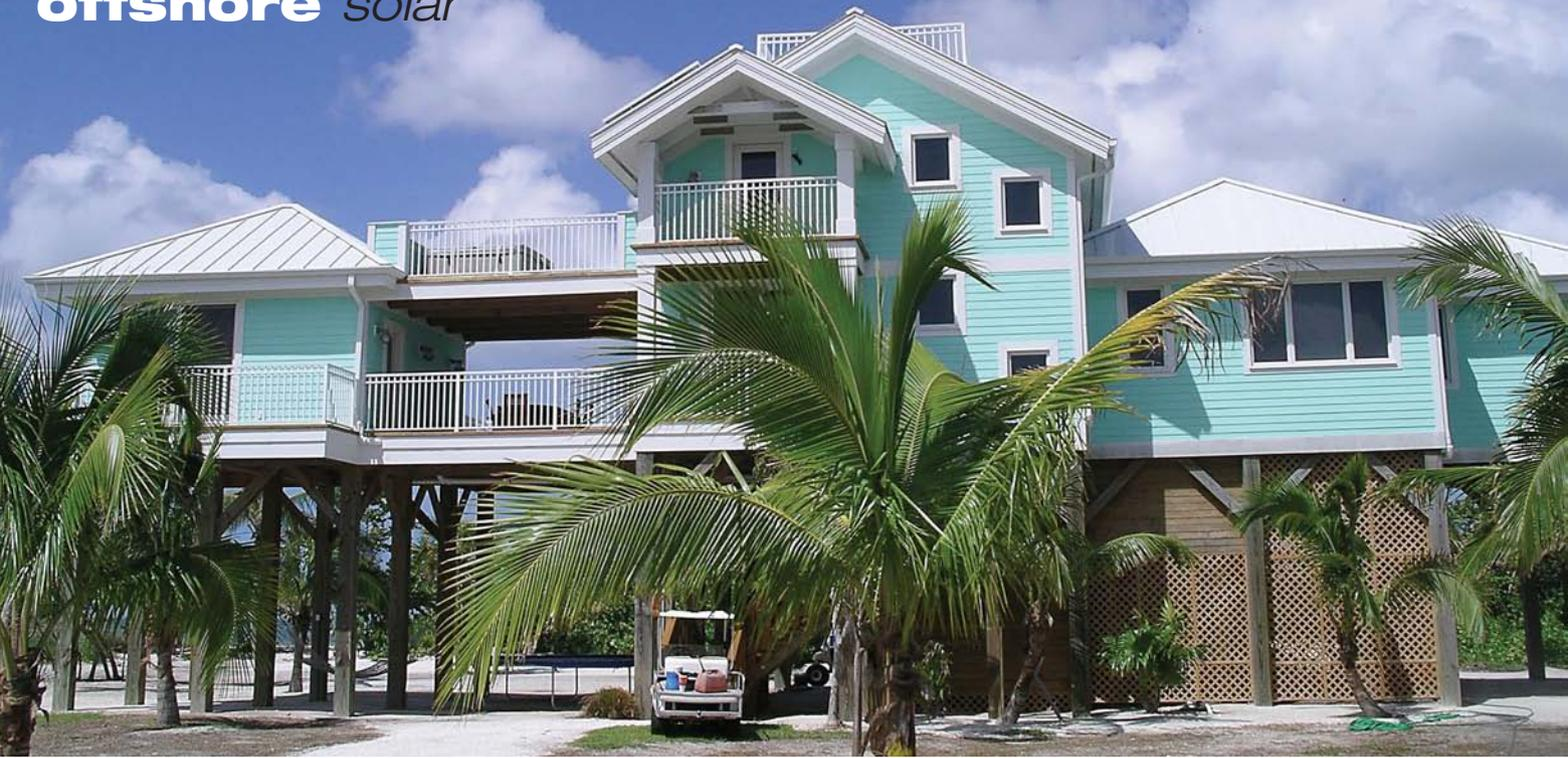
**Elevated to second-story level, the McVickers' house is designed to catch cool ocean breezes. Deep roof overhangs shade the windows and help their home keep cool.**
